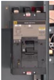
LAL36400 Tenant Circuit Breaker Supplied Factory Installed
