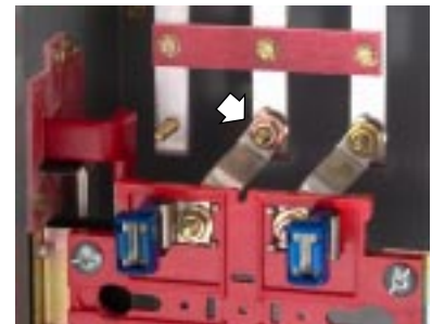
Step 6: Replace hex nut (removed in step one) onto stud of B \phi vertical bus and torque to 75 lb-in (8 N•m).
