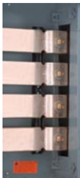
Shown After Installation of Cross Bus Structure is Completed
