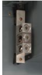
400 A Branch Unit Load Neutral Terminals
