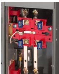
5-Jaw Kit (5J) Installed at the 9 O'clock Position
