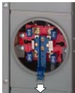
Manual Slider Type Bypass Shown in Closed Position with Handle Extending Through Notch in Rim of Meter Socket Trim
