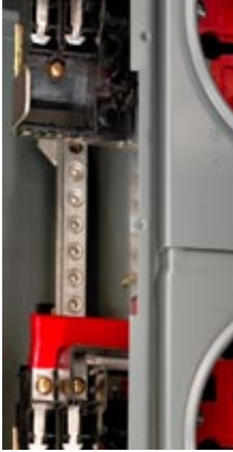
125 A Branch Unit Load Neutral Terminals
