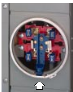
Manual Slider Type Bypass Shown in Open Position with Handle Secured by Meter Socket Sealing Ring
