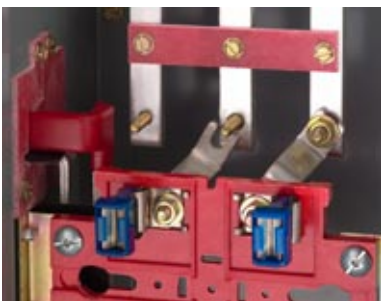
Step 3: Rotate "Z" connector to right and align with stud on B \phi vertical bus.
