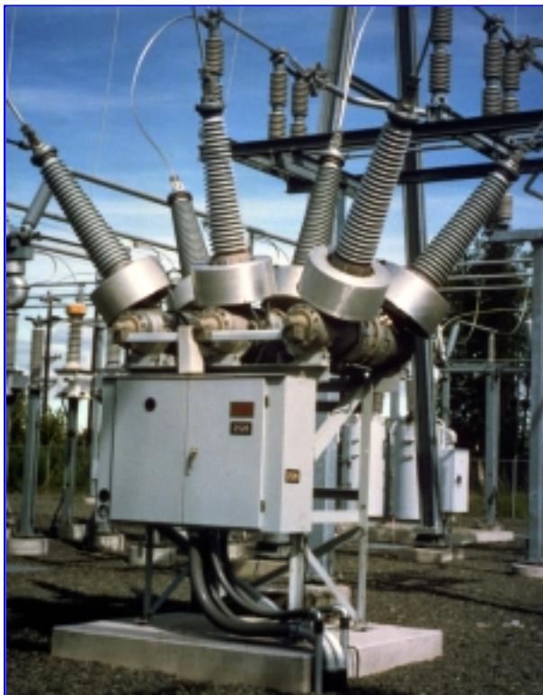
**The PM breaker is designed with components and experience gained through other quality ABB SF<sub>6</sub> breakers. This experience and the unequalled performance records of ABB breakers stands as a model for this design.**
